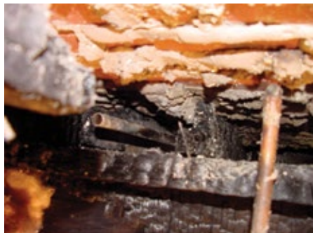
Charred wood inside a face wall after a house fire.
