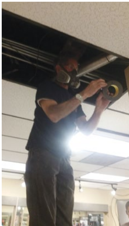
Frank Ayres taping the dryer exhaust duct after cleaning.
