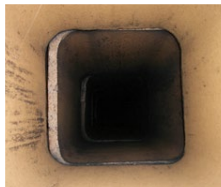
Gap between flue tiles.
