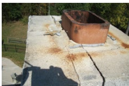
Cracked crown.
