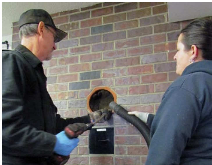
While using a foam plug to contain the soot, Scott sweeps while Hillary catches any stray dust with the vacuum.
