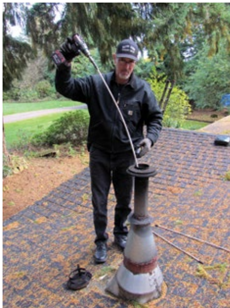
Scott rotary sweeping a pellet stove chimney.
