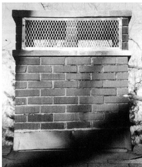
Stainless steel mesh used to screen an elevated slab chimney cap.
