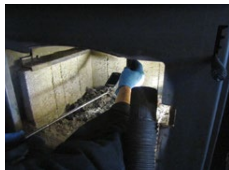
Checking the flue with a mirror from inside the stove.
